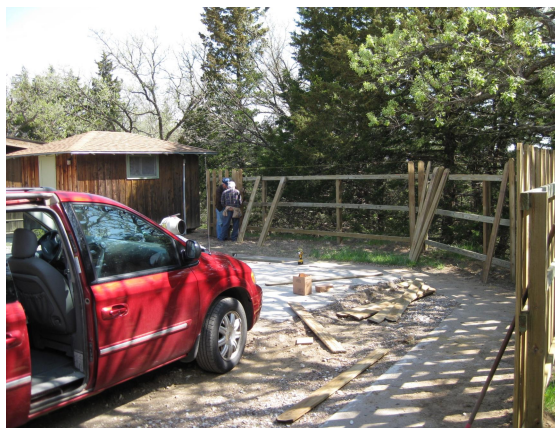
During Project Work Week in May, Stan Oberhelman, Chapman, and Dave Black, Holdrege, built a fence from Wiechelma to the Snack Shack.
